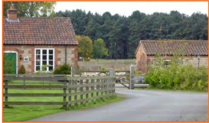
A good example of a conversion and refurbishment of a property at the Old Saw Mill
