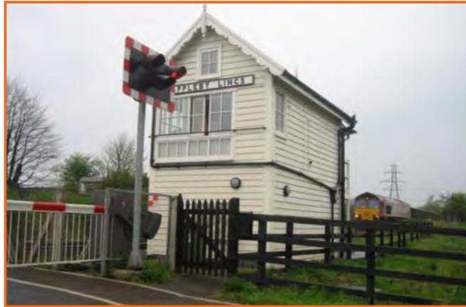
Appleby Level Crossing: the Signal Box is listed
